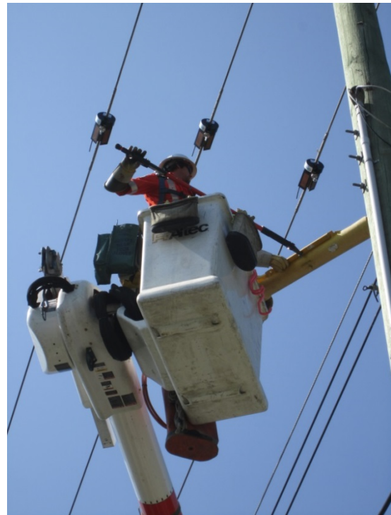
Figure 2: Sensors are easily installed with a hot stick on live MV lines.
